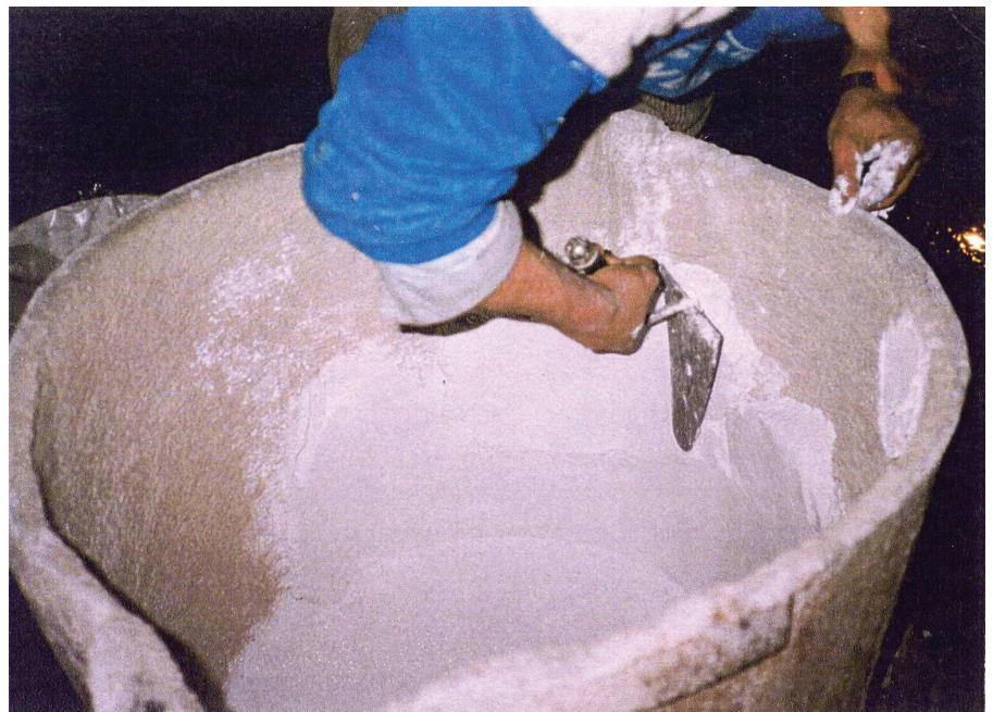
Pic 4: ISOPLAST PH 61 application by trowel
