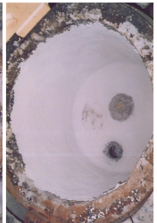
Pic 1: ISOPLAST PH 61 application completed
