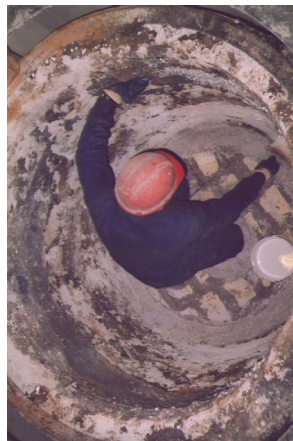
Pic 1: ISOPLAST PH 61 application by hand
