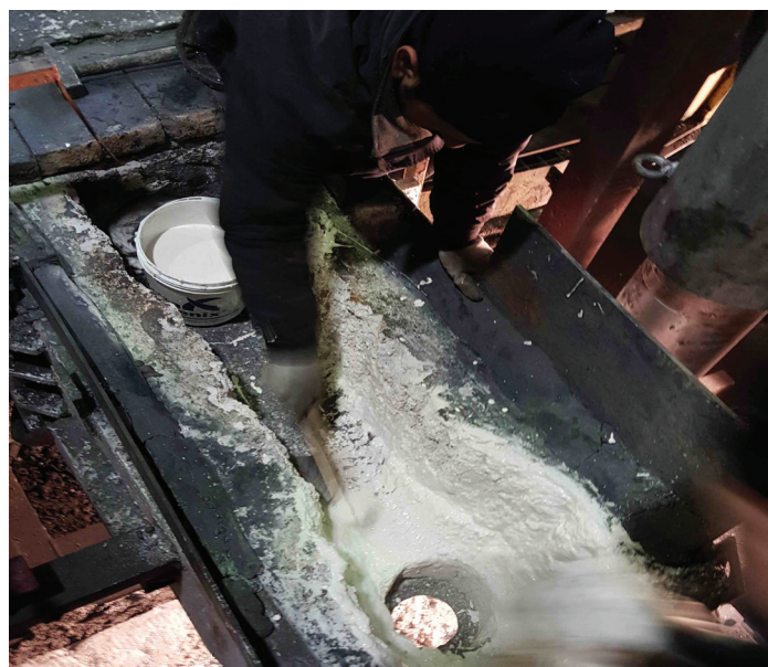
Picture 1: STUCK PH 10 application on pig-iron casting channels
